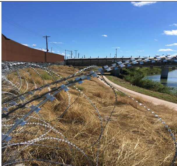
Figure 3. Concertina Wire Strapped to Bollard Fence, Brownsville, Texas, November 16, 2018
