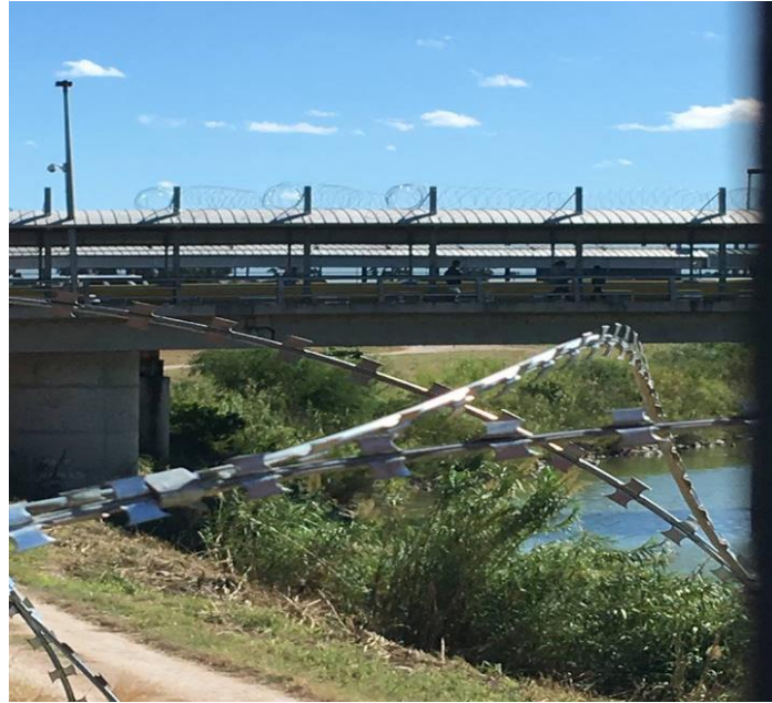
Figure 4. Gateway International Bridge, Brownsville, Texas with Concertina Wire Configured on Top of the Port of Entry
