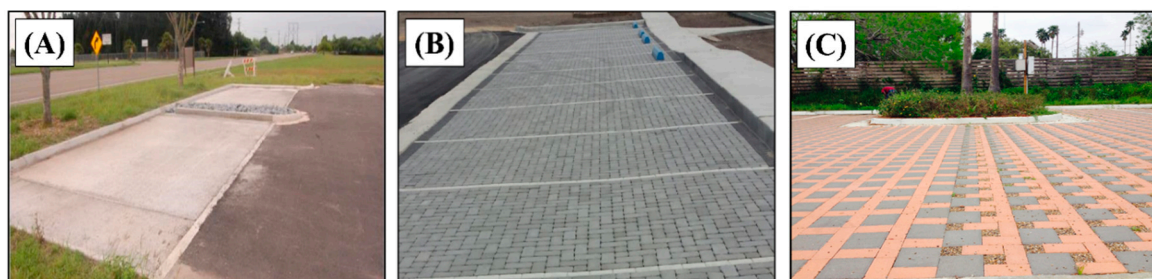
Figure 1. Three types of monitored permeable pavements in different parking lots at Lower Rio Grande Valley (LRGV) sites. From the left: (A) Porous Concrete Pavement (PCP), (B) Permeable Interlocking Concrete Pavement (PICP), and (C) Interlocking Block Pavement with Gravel (IBPG).
