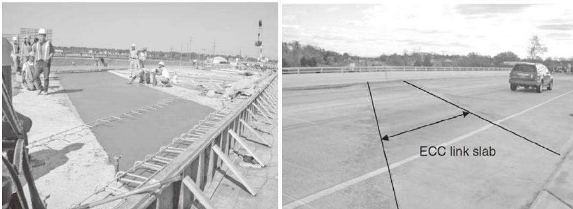
Figure 5-4 ECC Link Slab Constructed in Michigan (Li 2014)
