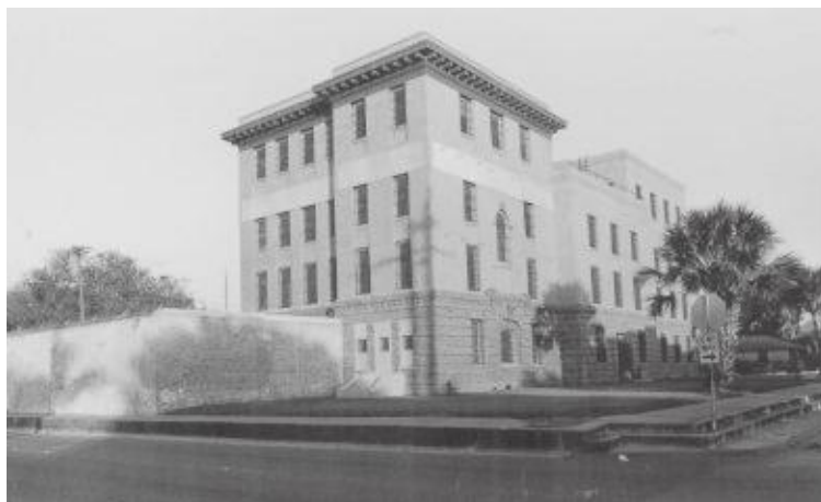
Old Cameron County Jail
