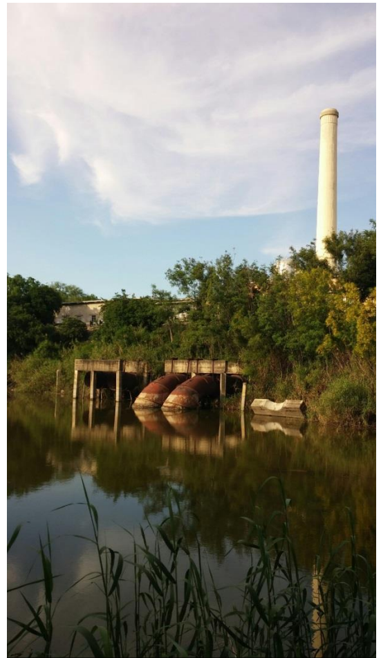
Figure 5: Pumps at irrigation system headwaters. A canal had to be dug to the spot after a massive hurricane in 1933 shifted the course of the Rio Grande. (Photo: Aaron Cummings)
