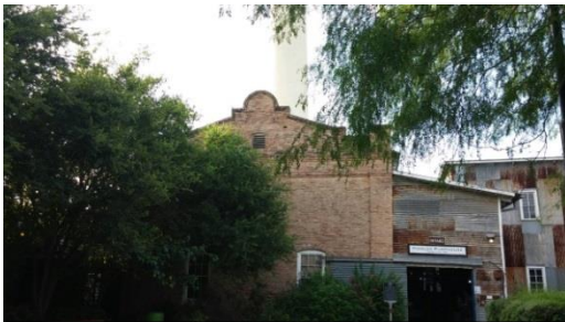
Figure 4: Hidalgo Pump House, built 1909 (Photo: Aaron Cummings)
