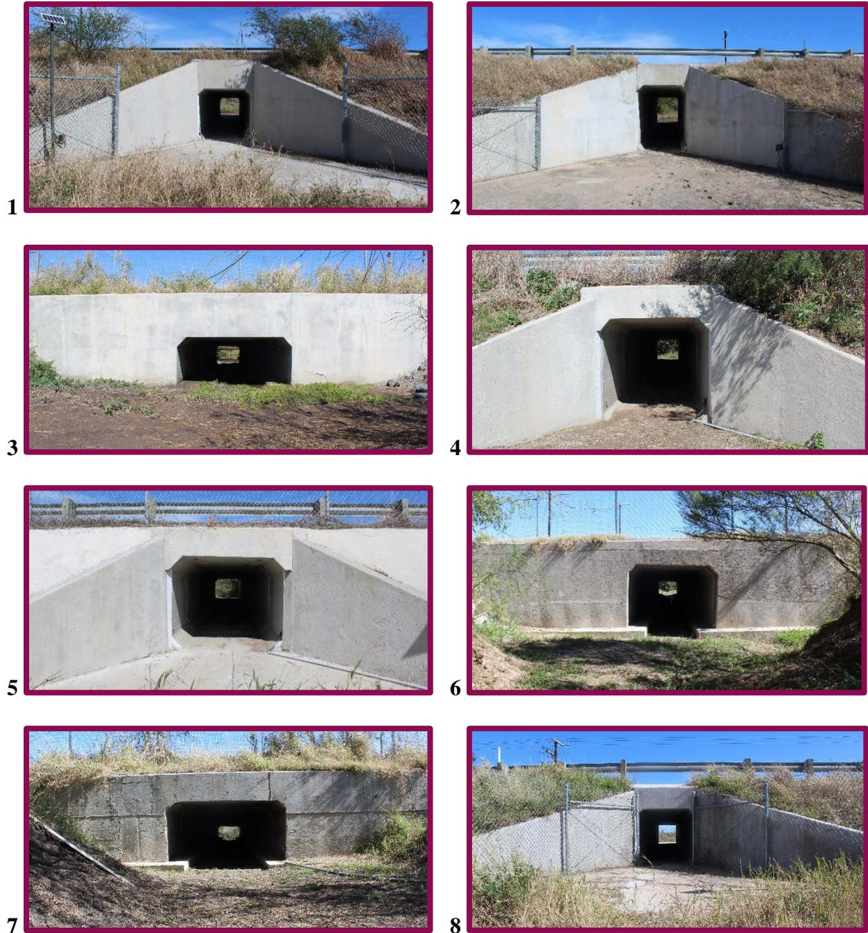
**Figure 3.** Eight wildlife crossing structures (WCS) were installed under Farm to Market Road (FM)106 in Cameron County, Texas. From top left, they are referred to as WCS 1 - 8. WCS 3 experiences regular sediment infill and flooding and as such is monitored with a fully passive infrared (PIR) camera trap system rather than a partially active infrared (AIR) system.
