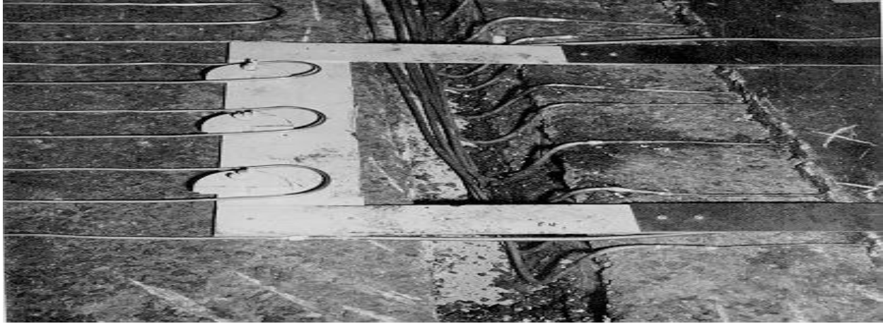
Figure 5: Electric cables in the bridge approach roadway, Newark, New Jersey 1961 [25]
