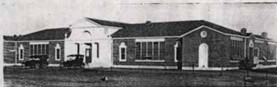
Sharyland High School and Grade School
